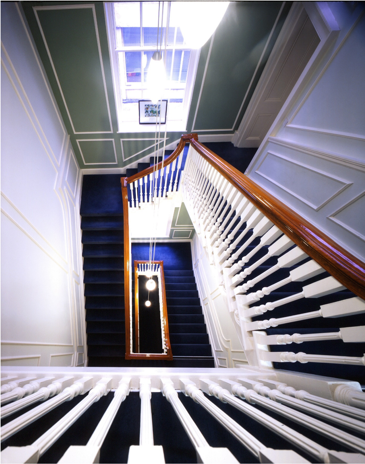
H. Square staircase (from the top)
